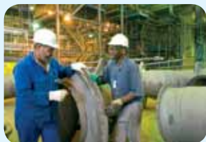
Restoration work at Komati power station
